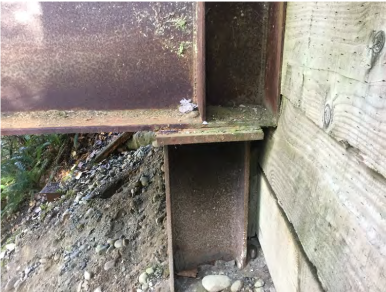
Downstream Left bank bearing
