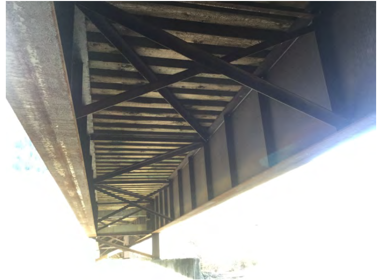
Left span superstructure
