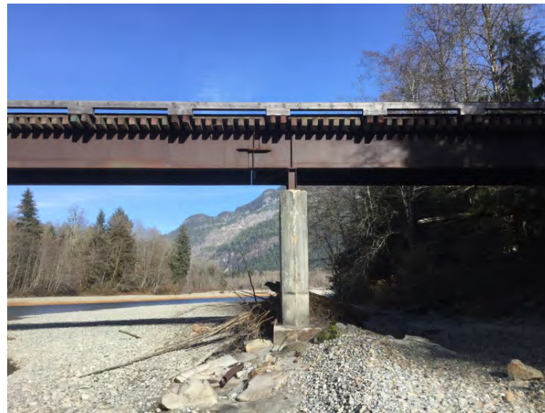
Left Pier and girder connection
