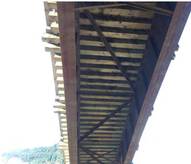
Span 2 from left bank superstructure
