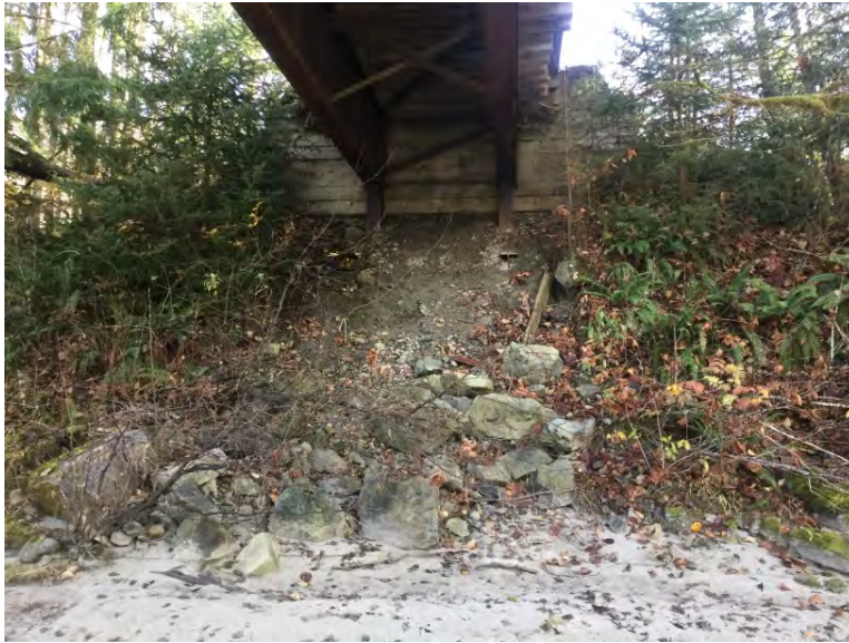
Left Bank Abutment when facing downstream
