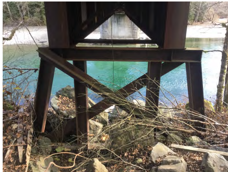
Pier 3 from left bank
