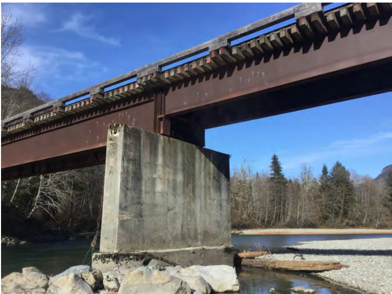
Span 2 from left bank at Pier 2
